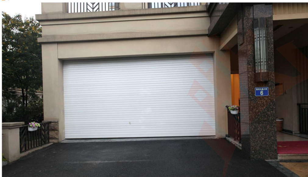
★ 铝合金卷帘车库门在广州保利城安装案例 ★ Aluminum alloy shutter garage door in Guangzhou poly City installation case
