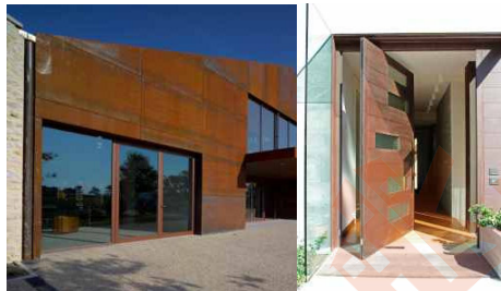
Corten steel doors
